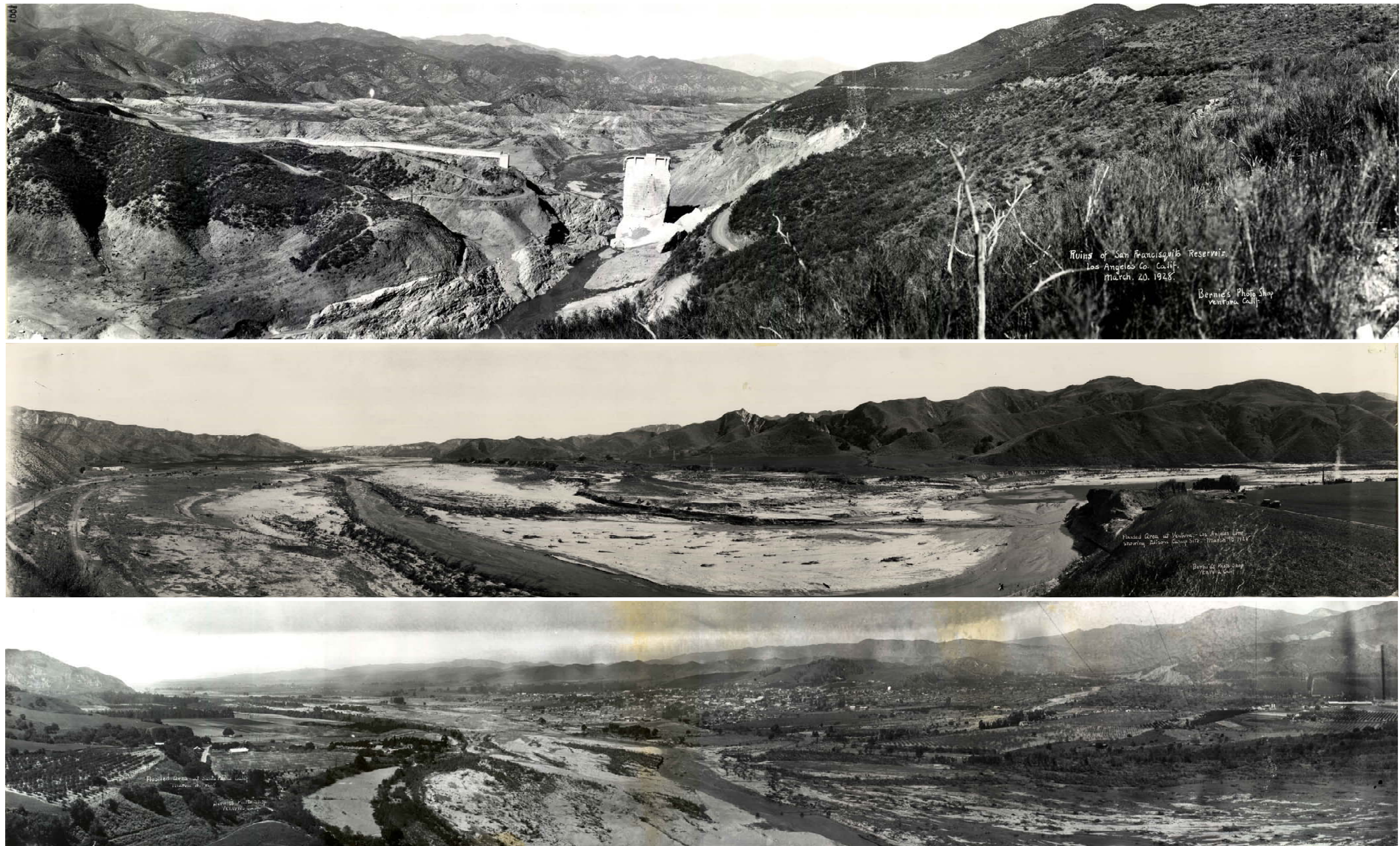
Figure 4-7. The remains of the St. Francis Dam after collapsing just before midnight on March 12, 1928, in the San Francisquito Canyon subwatershed (top). Middle, a downstream view of the mainstem Santa Clara River near the County line, five days after the dam break flood. Below, a downstream view of the mainstem SCR near Santa Paula Creek, the day after the dam break flood. Photos courtesy of the VCWPD.
