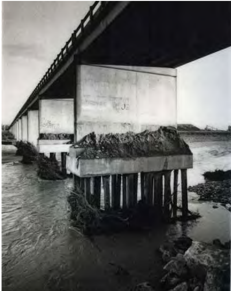
Figure 4-9. Undercutting of the Highway 118 bridge over the SCR as a result of incision following the 1969 floods. (Photo courtesy of the VCWPD.)
